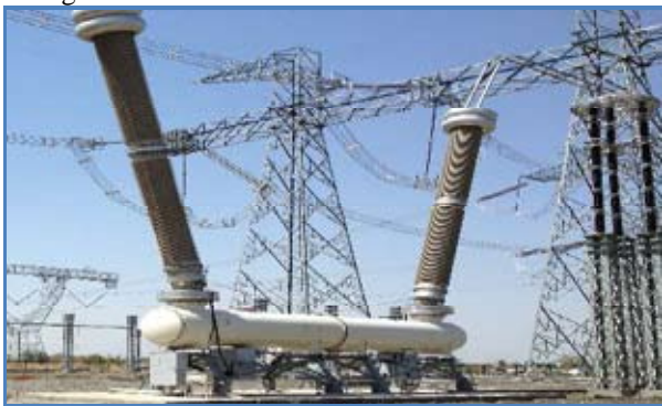
Fig. 1(c): 1200 kV Dead tank breaker
